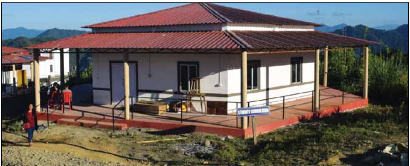
Mizoram Engineering College, Date of Completion : 16.11.2018 Location: Arsi Ram Pukpui, Lunglei District, Lunglei, Mizoram Pin No.796701
