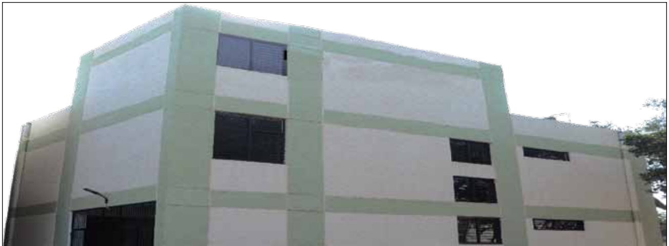
Smart Class & Laboratory M N College, Visanagar, Gujarat, Date of Completion : 09.09.2018 Location Manekalal Nanchand College Visanagar, Near Bus Staton At & PO – Visanagar-384315 Date of Picture taken : 09.01.2019
